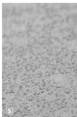
Matt stone structure
